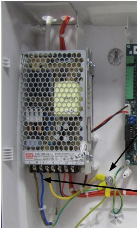
Figure 20 Connecting Mains AC power
